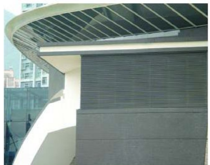
Indoor Recreation Centre, Ma On Shan, Hong Kong. Universal Louvre for plant room ventilation and for controllable air inlet for the smoke extraction system.
